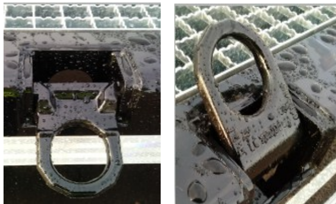
Figure 23: Example of Lashing Ring
